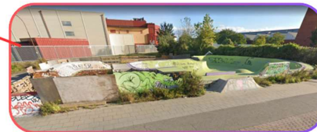
Pig Barrier DIY skatepark i betong Industrigatan 22, 212 14 Malmö.
